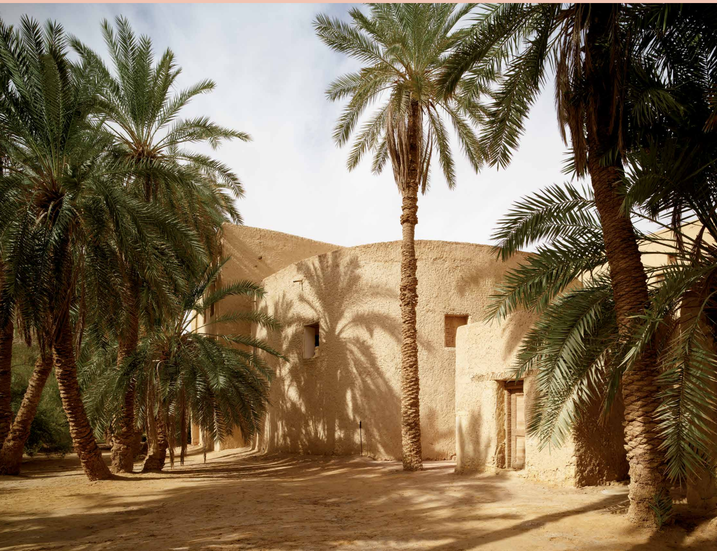
Tamazid's entrance, like the rest of the building, was constructed with kershef , a traditional building material made from mud and salt. Opposite: a shaded balcony features a stone sculpture designed by the Chinese artist Li Shuang and executed by a local sculptor. The windows were placed strategically to catch prevailing breezes.
